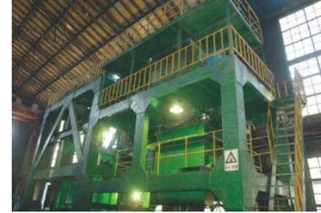
Vibratory compaction machine.
